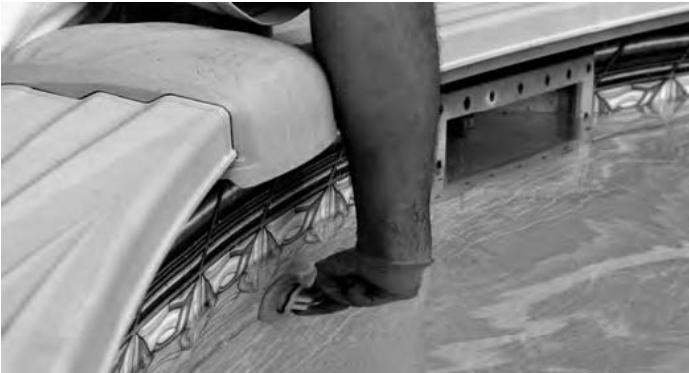
5. **Make sure the filter pump is turned OFF** so no water flows out of the filter when disconnecting the return hose from the swimming pool return Inlet.
